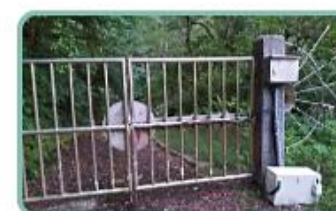
實體電子圍籬 (磁簧式) Physical electronic fence (reed type)
